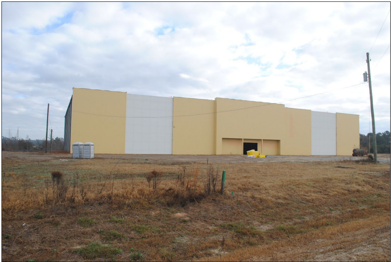
Figure 3.6 View of disturbed area and newly constructed building, facing east.
