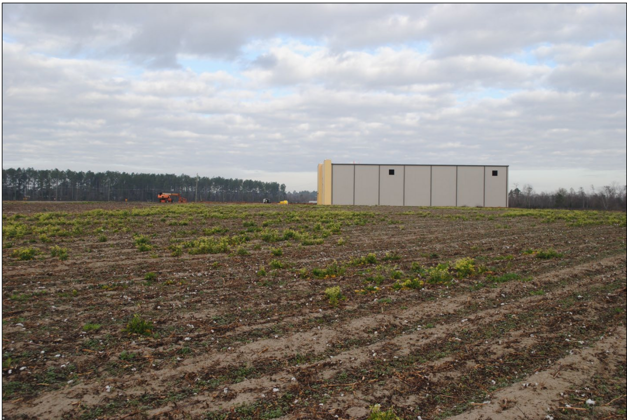
Figure 3.5 Typical view of the project tract facing new building, facing east.
