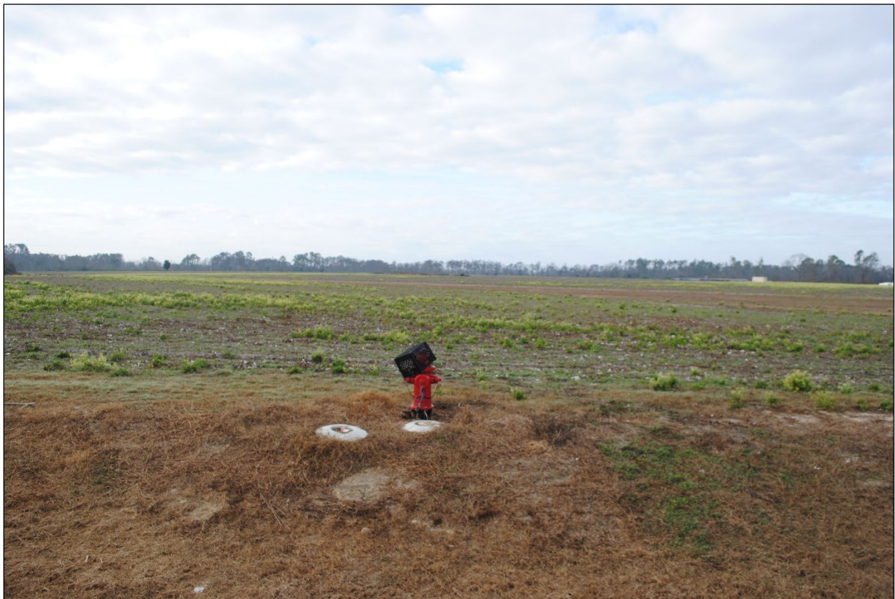
Figure 3.7 View of project tract and buried waterline, facing southwest.
